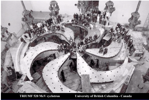
Cyclotron (H - accelerated, protons extracted)
